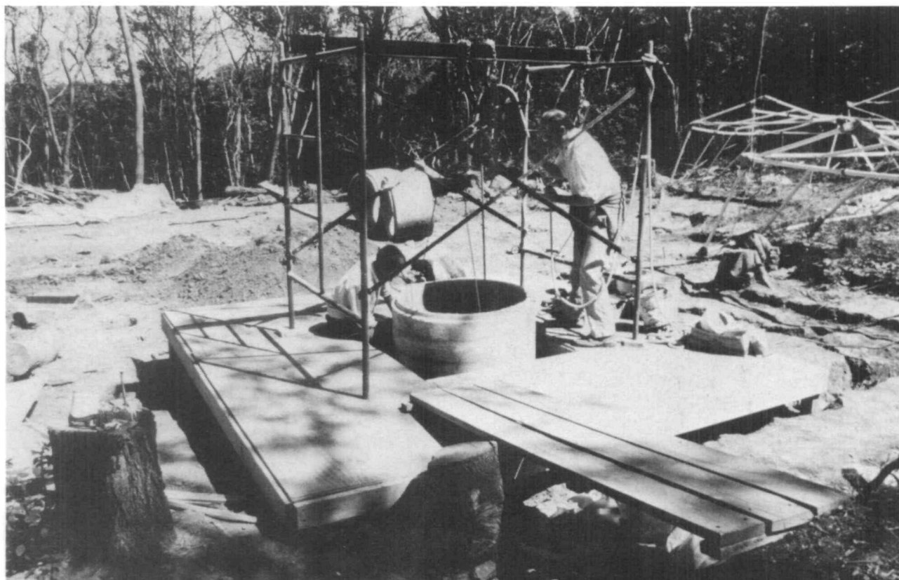
FIGURE 6. Area I Well Excavation, Illustrating Platform Scaffolding, and Concrete Well Rings in Place.
