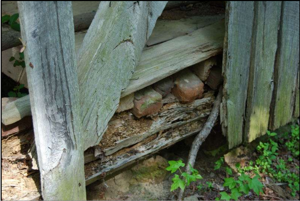
Figure 18. Handmade bricks used in the construction of the corn crib.
