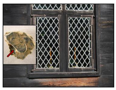
**Figure 20.** Window glass (shown with arrow) still encased by glass window frame (inset). Reconstructed window, Farthing's Ordinary, Historic St. Mary's City.
